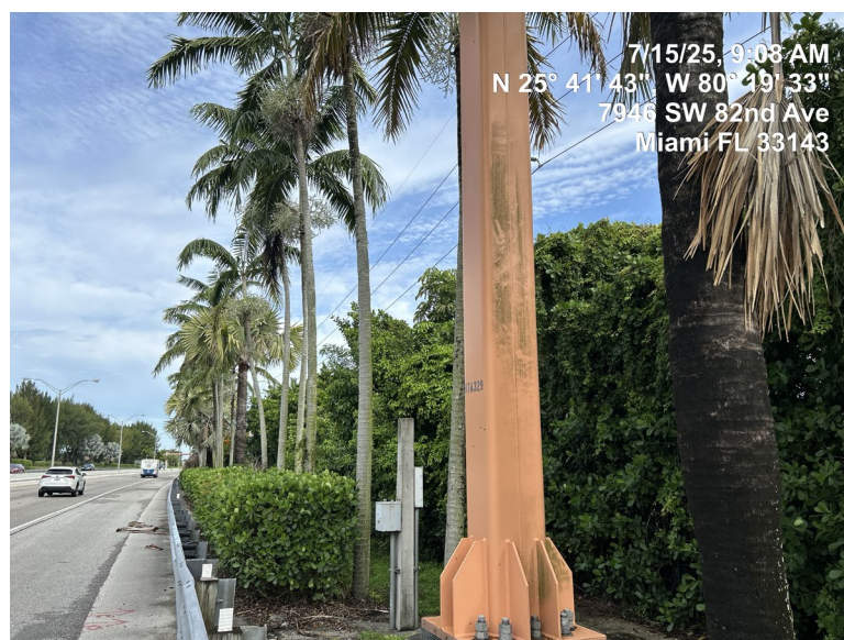
DETERIORATED PAINT ON DMS SIGN STRUCTURE (STRUCTURE #87A329)
